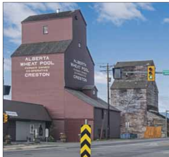
The Alberta Wheat Pool elevator in Creston, B.C., has been restored. The elevator beside it isn't in as good of shape.
