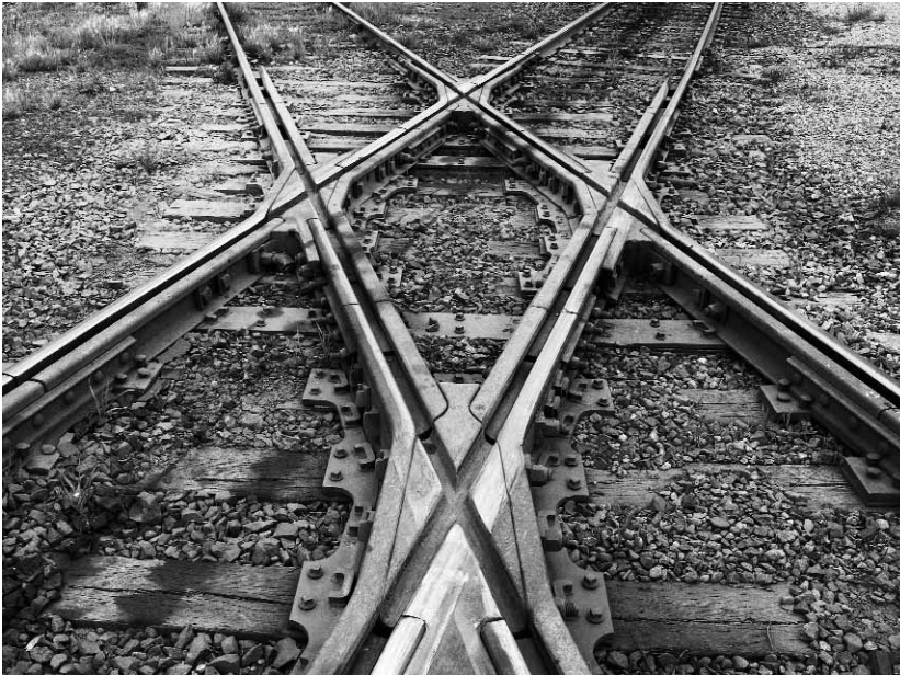
Railway tracks at the Diamond Intersection.
